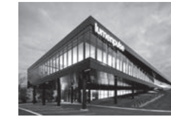
Lumenpulse Headquarters Longueuil, Quebec, Canada Architect: Lemay Photographer: Stéphane Brügger
