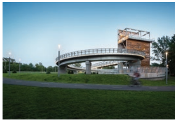
Passerelle Normandie Longueuil, Quebec, Canada Architect: Cardin Julien Engineer: CIMA + Photographer: Steve Montpetit
