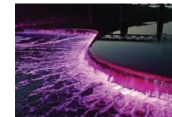
Grand River Penman's Dam Portage Paris, Ontario, Canada Lighting Designer: Mulvey+Banani International Inc. Photographer: Joel Batters
