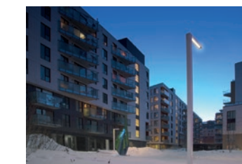
Arbora Griffintown Montreal, Quebec, Canada Architect: Lemay Photographer: Leigh Gice
