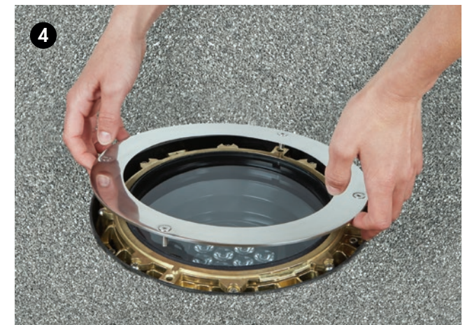
4 Put the stainless steel trim in place.
