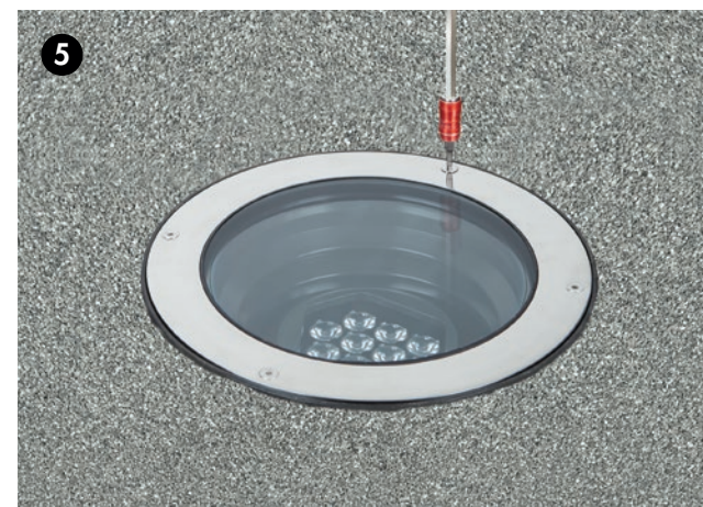
5 Lock the trim in place using the appropriate driver.
