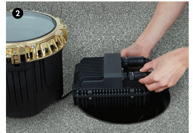
2 Plug the luminaire into the PCBX.
