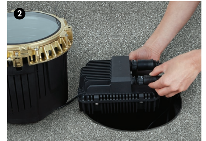
2 Plug the luminaire into the PCBX.
