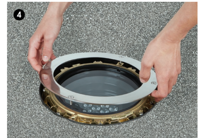
4 Put the stainless steel trim in place.
