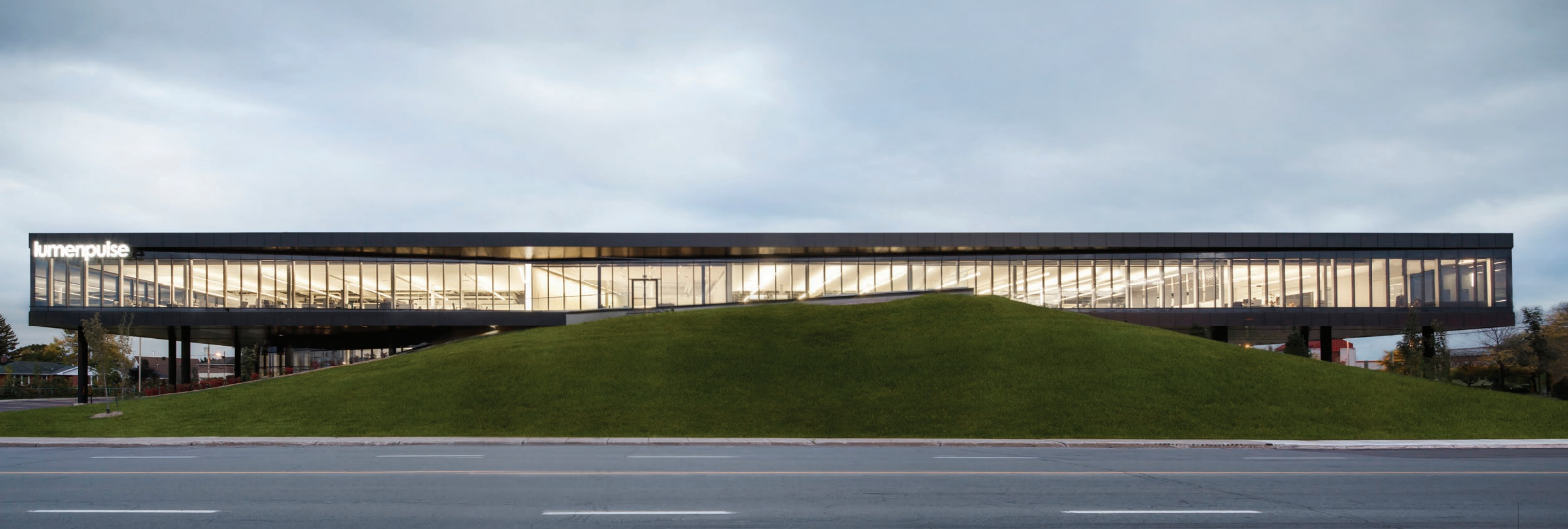
Lumenpulse Headquarters Longueuil, Quebec, Canada Architect: Lemay Photographer: Stéphane Brügger
