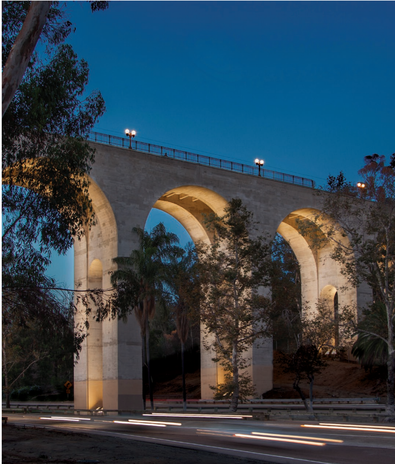
Cabrillo Bridge San Diego, California, United States Lighting Design: Illumination Arts Photographer: Steve Lerum
