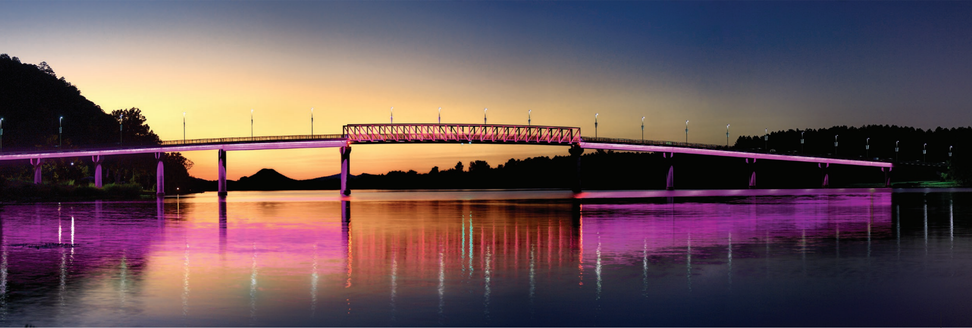
Two Rivers Park Bridge Little Rock, Arkansas, United States Engineer: Garver LLC Photographer: Mike Anderson
