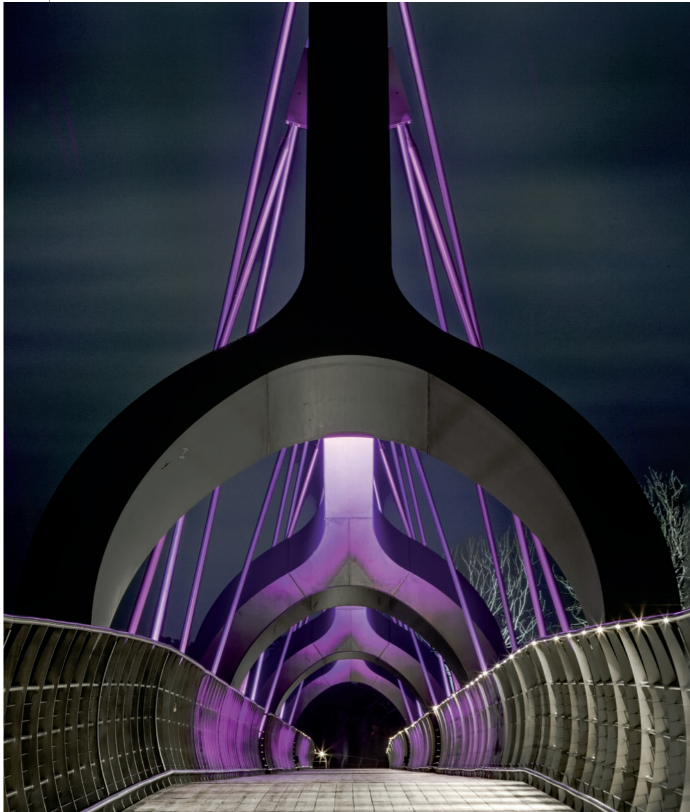
Sölvesborg Bridge Sölvesborg, Sweden Lighting Design: Ljusarkitektur Photographer: Olof Thiel
