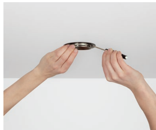
2 Unclip the Lumencore from its ceiling mount.
